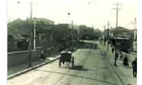
2 Marrickville Shopping Centre, Illawarra Road (c1936)
