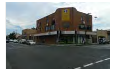
② Corner Victoria and Sydenham Roads
